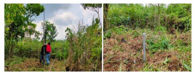
Figure 9. The installation of 4 units of piezometers at FC 25 and 38 of Bukit Belata (Ext.) Forest Reserve
